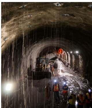
Tunnel Garage Côte-Vertu – excavation
