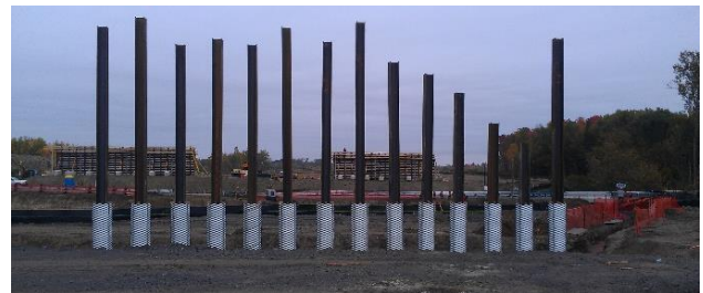
Figure 14. Installation of corrugated steel pipes
