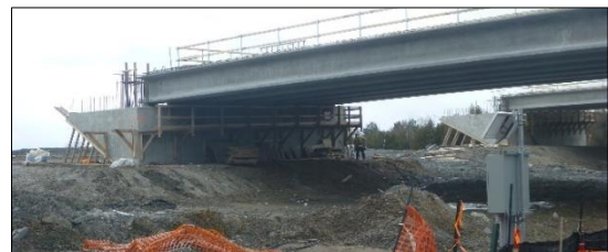
Figure 12. Northbound lane of the south abutment
